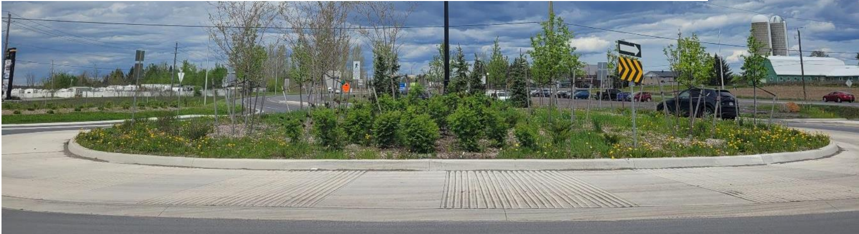
Example: Limoges Road (County Road 5) at Route 300, Russel Township, United Counties of Prescott and Russell, ON
